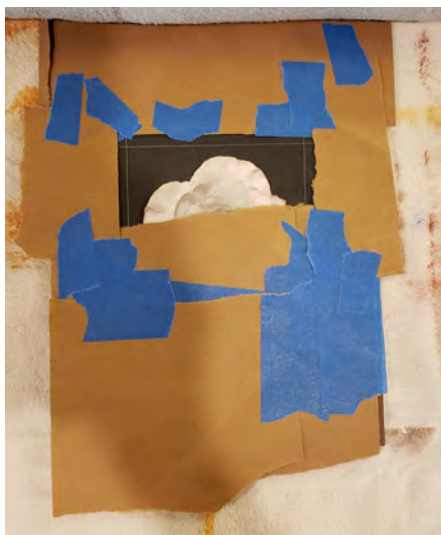
Photo 9: Protect from overspray
